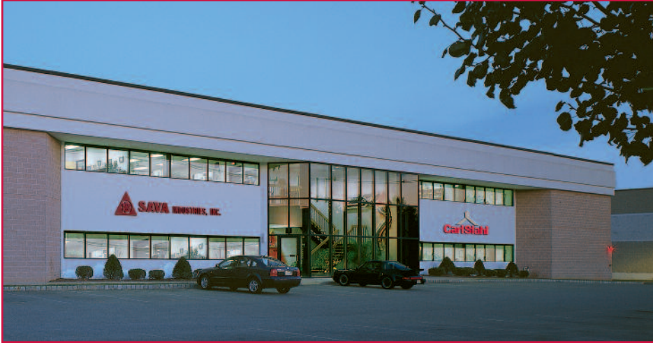
Carl Stahl Sava Industries Headquarters and Manufacturing Facility in Riverdale, NJ
